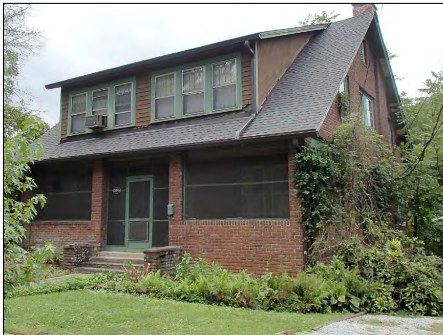
Figure 57: Masonry, side-gable bungalow, 301 Maple Street
