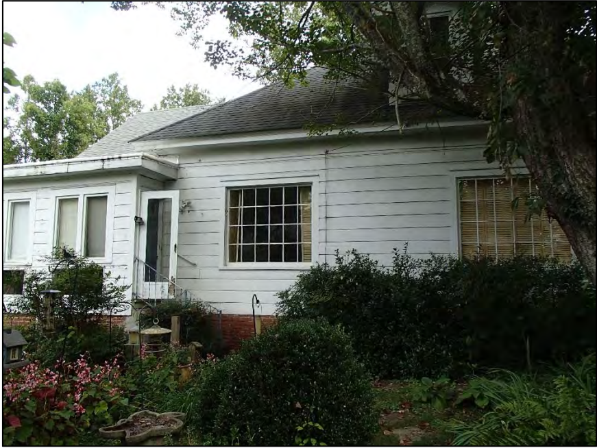
Figure 96: Vassey-Caldwell House, southwest elevation
