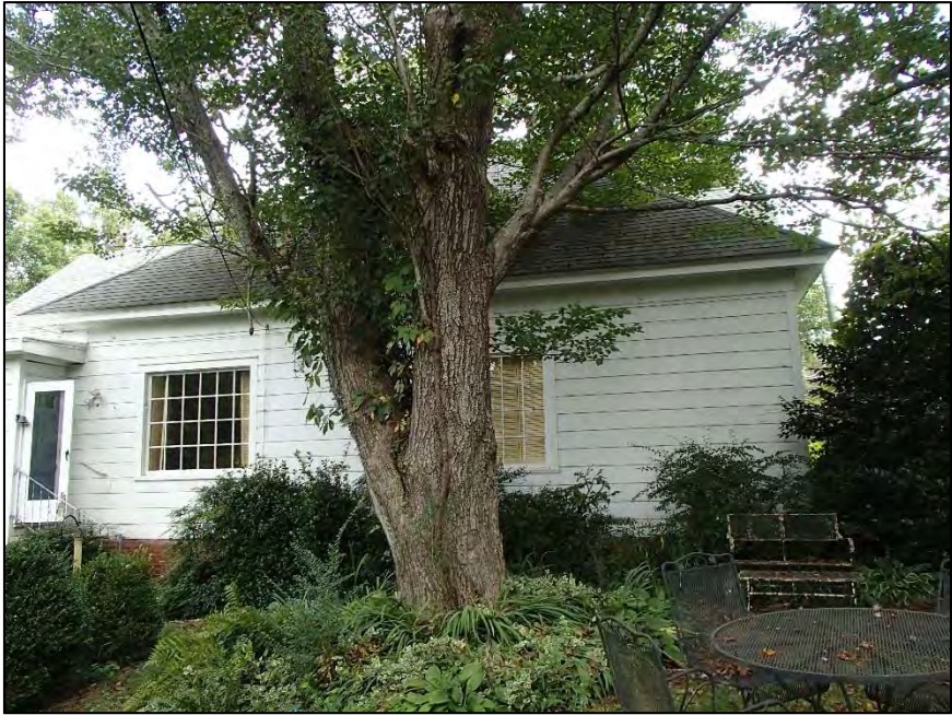
Figure 97: Vassey-Caldwell House, southwest elevation
