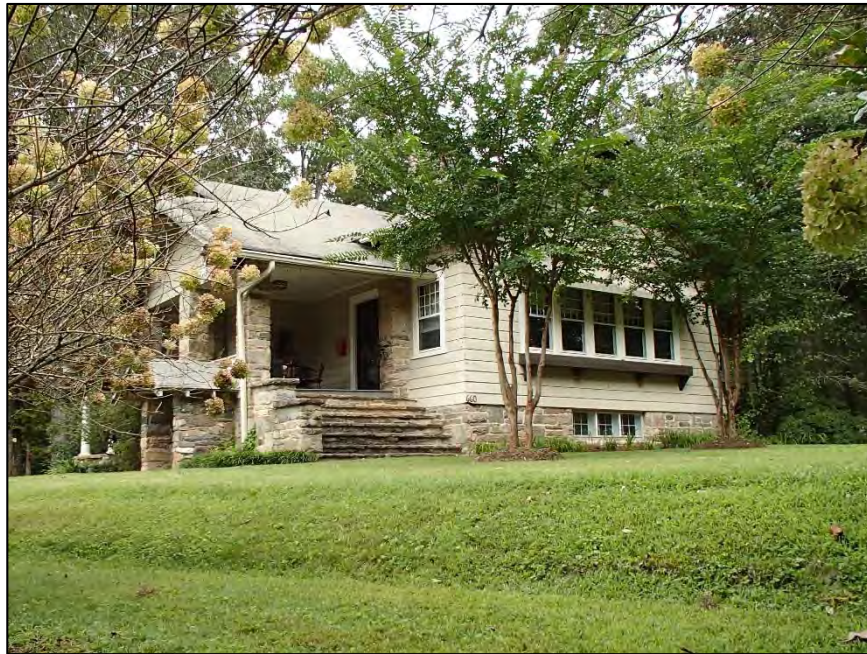
Figure 56: Carrie-Plummer House, 660 East Main Street
