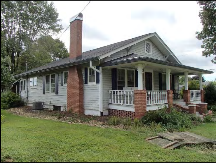
Figure 67: DeBord Family House, northwest corner
