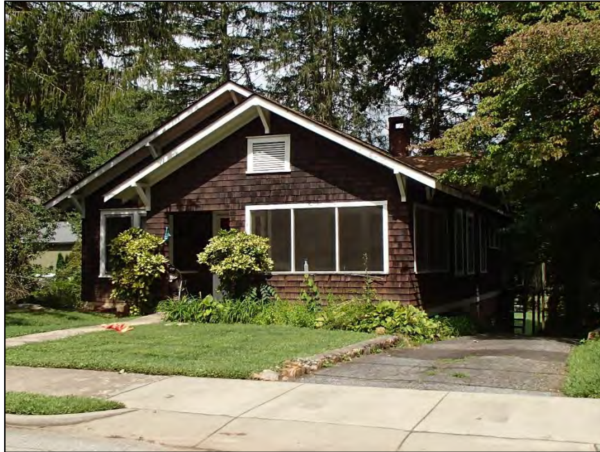
Figure 72: Gable-front, shingled bungalow at 191 Park Avenue
