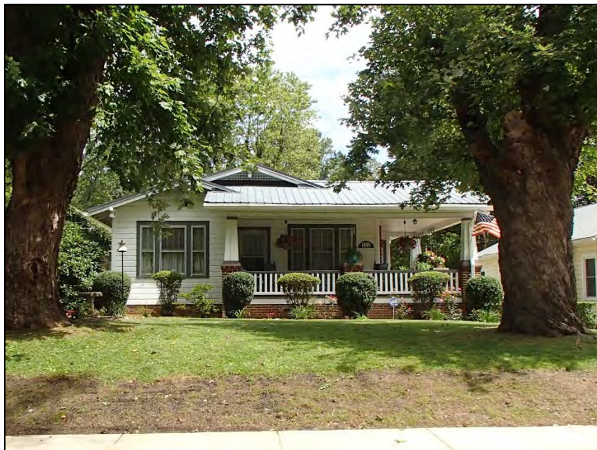
Figure 74: Gable-front bungalow with side-gable porch, original windows, and drop siding at 121 Maple Street
