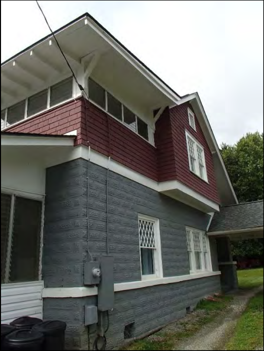
Figure 49: Osborne-McCormick House, north elevation
