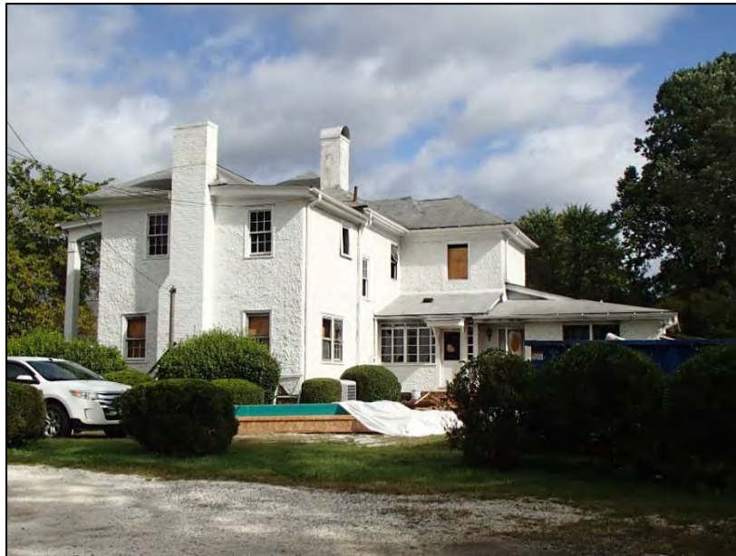
Figure 30: Robinson-Newland House, south elevation
