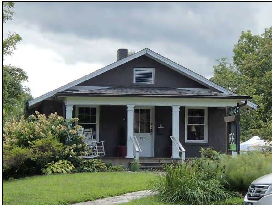
Figure 39: Bungalow at 173 West Main Street
