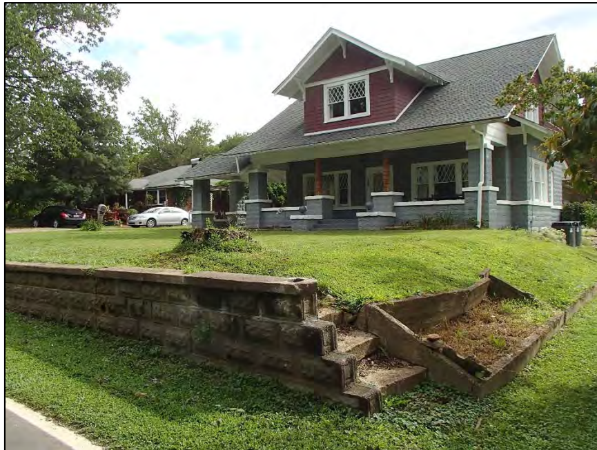
Figure 45: Osborne-McCormick House, southwest corner and retaining wall
