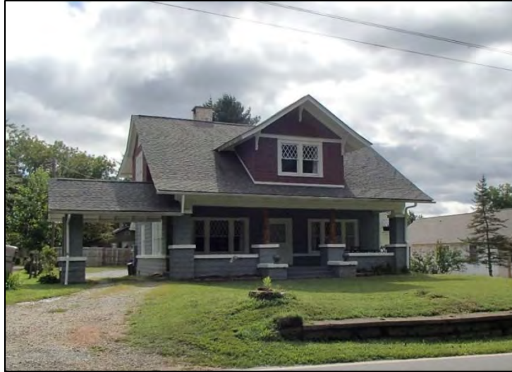
Figure 50: Osborne-McCormick House, west elevation
