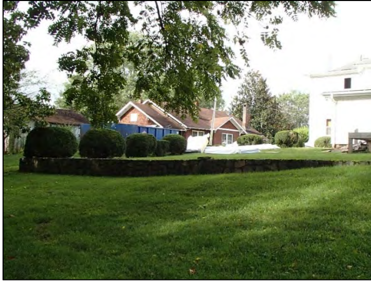
Figure 31: Robinson-Newland House, rear retaining wall
