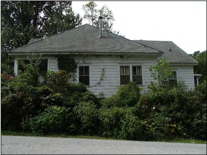
Figure 94: Vassey-Caldwell House, northeast elevation
