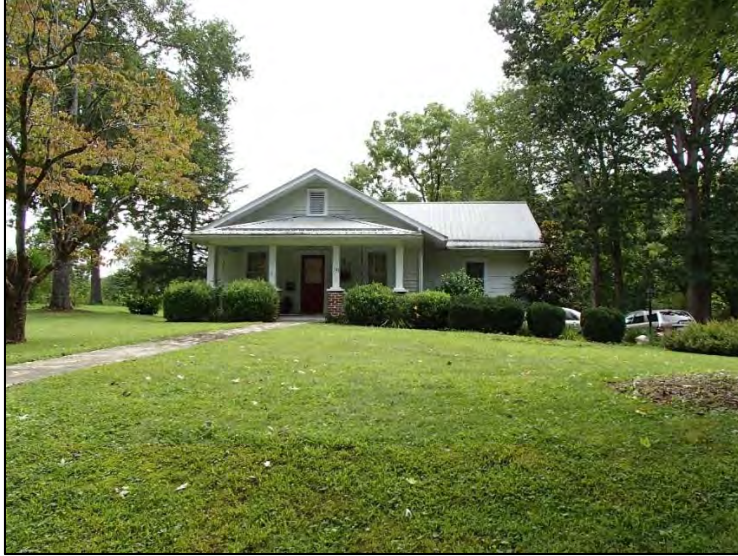
Figure 71: Gable-front bungalow with original weatherboards and shingles at 190 Parkview Drive
