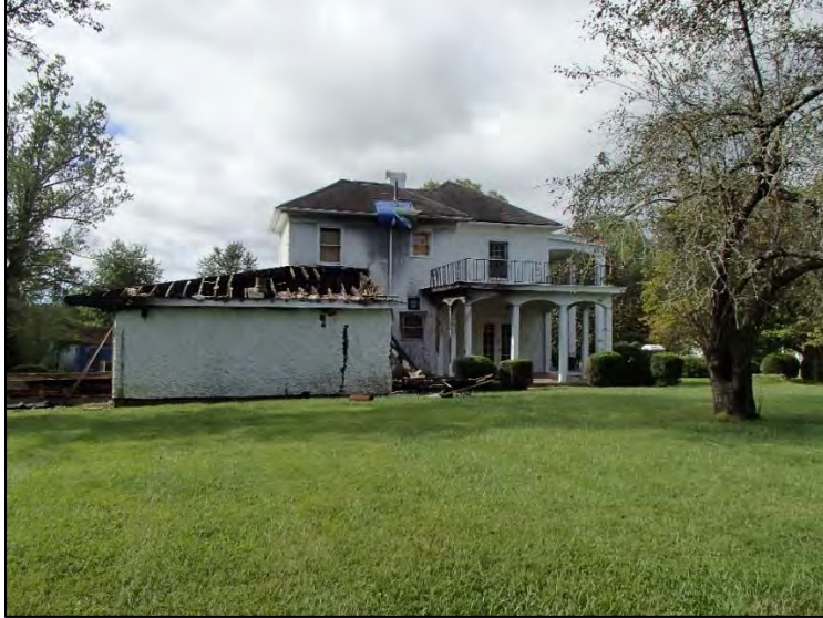
Figure 27: Robinson-Newland House, north elevation
