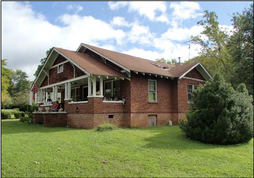
Figure 34: John and Tasrie Bishop House, southwest elevation
