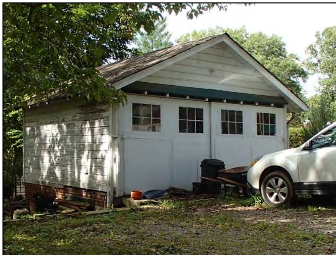
Figure 84: Miriam and Albert Kyle House, garage, north elevation
