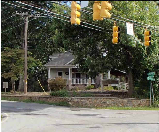
Figure 16: Rufty House, southwest elevation
