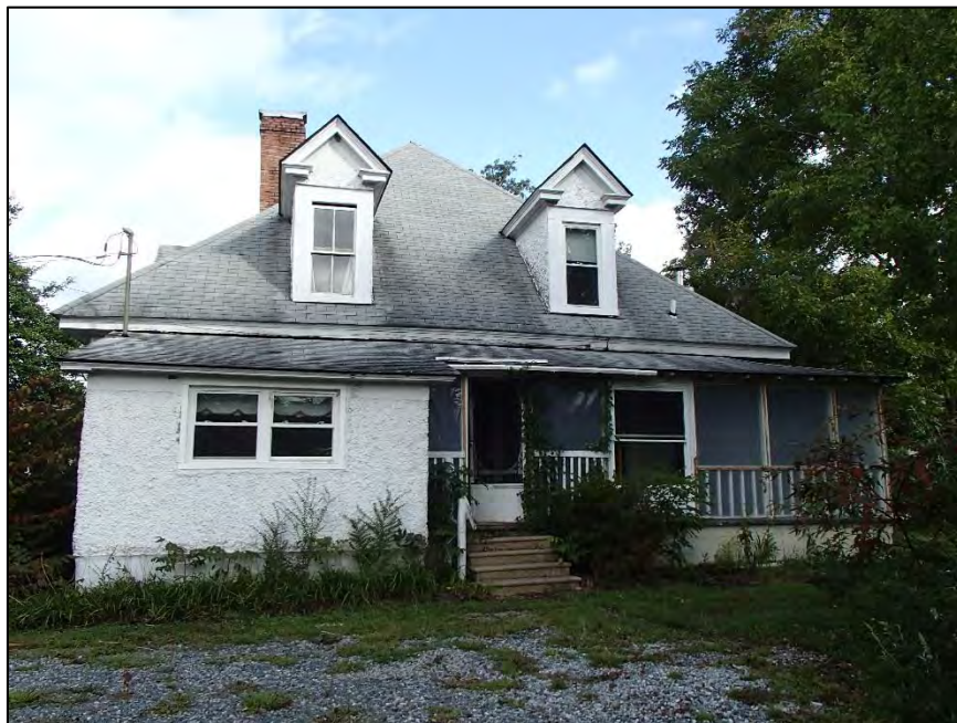
Figure 6: Louise Erwin Lewis House, south elevation
