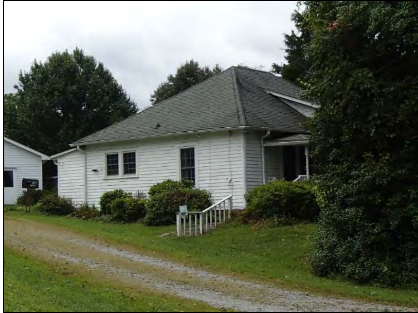
Figure 98: Unsurveyed cottage at 158 Old U.S. Highway 64
