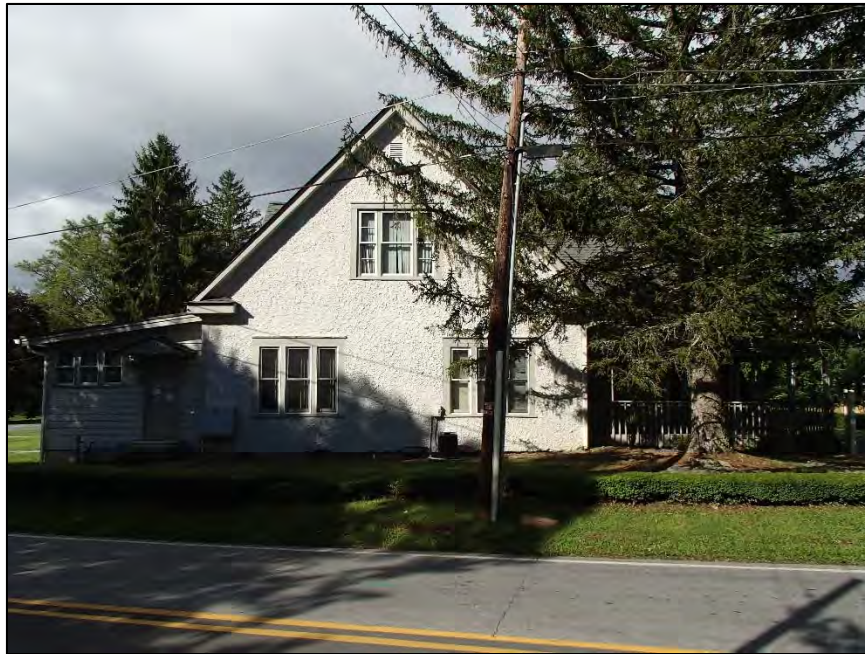
Figure 9: C. C. Younge House, east elevation
