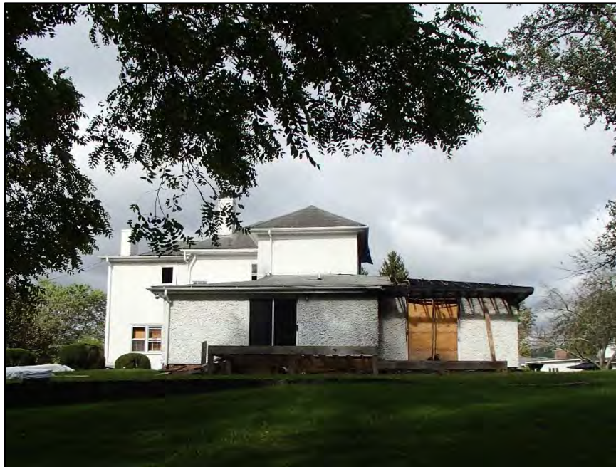
Figure 28: Robinson-Newland House, east elevation
