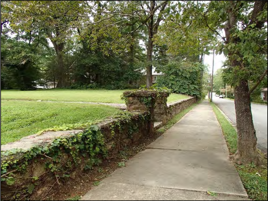
Figure 24: Rock wall along East Main Street, typical example of retaining walls throughout Brevard
