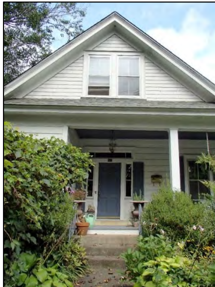
Figure 93: Vassey-Caldwell House, southeast elevation detail
