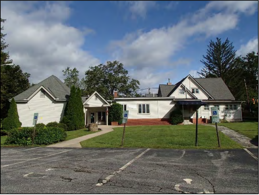
Figure 10: C. C. Younge House, south elevation
