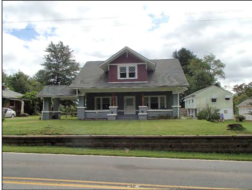
Figure 46: Osborne-McCormick House, west elevation
