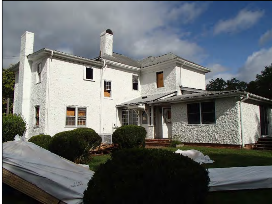
Figure 29: Robinson-Newland House, east elevation
