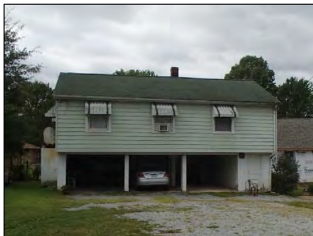
Figure 51: Osborne-McCormick House, garage apartment, north elevation
