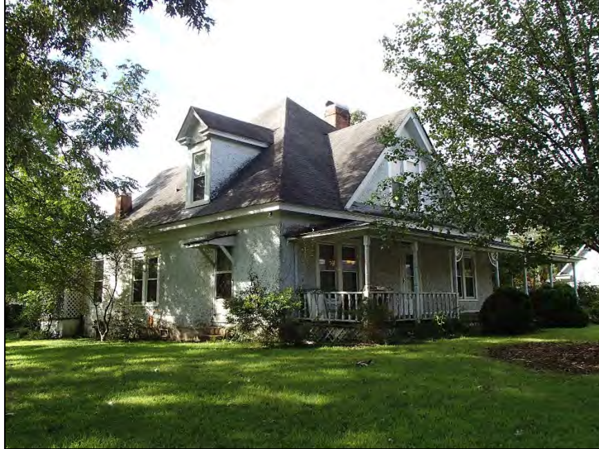
Figure 5: Louise Erwin Lewis House, northeast corner
