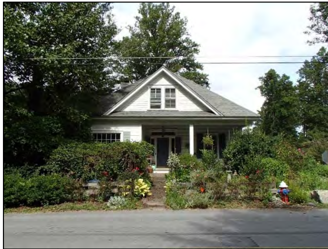
Figure 92: Vassey-Caldwell House, southeast elevation
